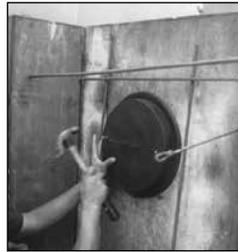
3. Place the CENTURY-LINE® Sleeve on the end cap. When field cutting non standard CS sleeve lengths, the sleeve and end caps total length should be 1/4" longer than the thickness of the wall. Cut with a hand or power saw.
