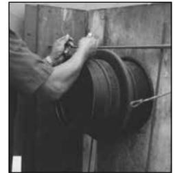
6. After the concrete is poured and cured, remove end caps with screw driver or crow bar. End caps may be replaced to protect sleeve until pipe penetration is made.
